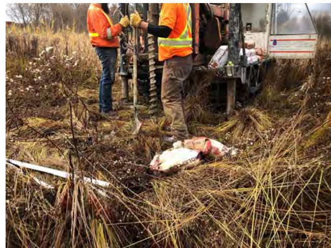
Photo 28: Abandonment of monitoring well OW6 (October 2019)
