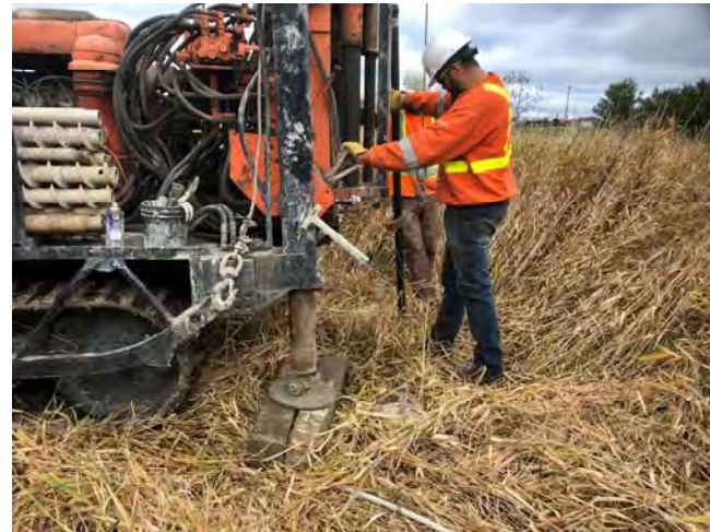
Photo 26: Abandonment of monitoring well L8 (October 2019)
