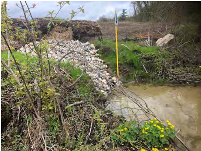
Photo 31: Tile drain discharge improvements near SW1 (October 2019)
