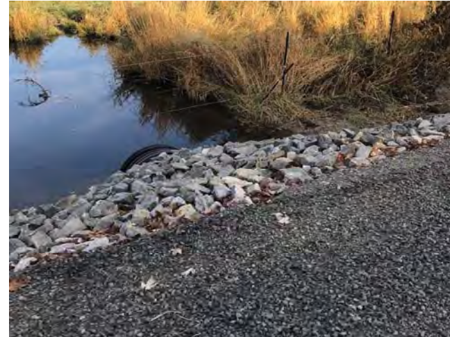
Photo 30: culvert improvements at SW5 (October 2019)
