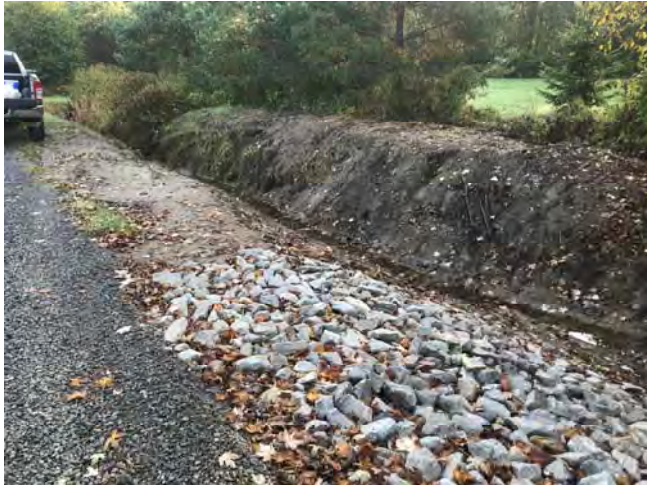
Photo 29: culvert improvements at SW5 (October 2019)
