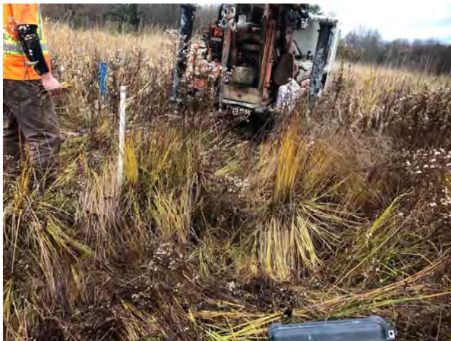
Photo 27: Abandonment of monitoring well OW7 (October 2019)
