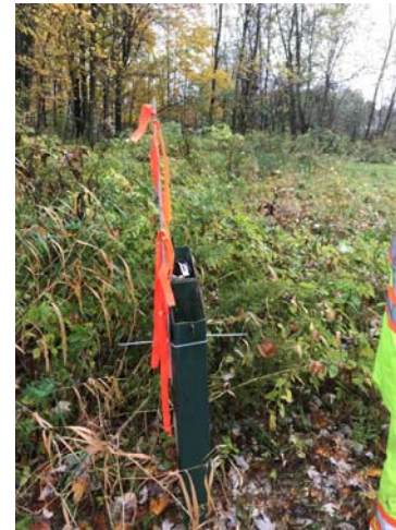
Photo 18: monitoring well OW24 (October 2020)
