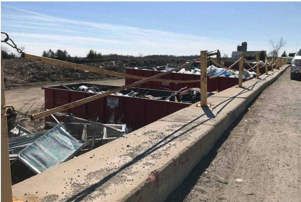
Photo 4: View of the waste bins and transfer facility.
