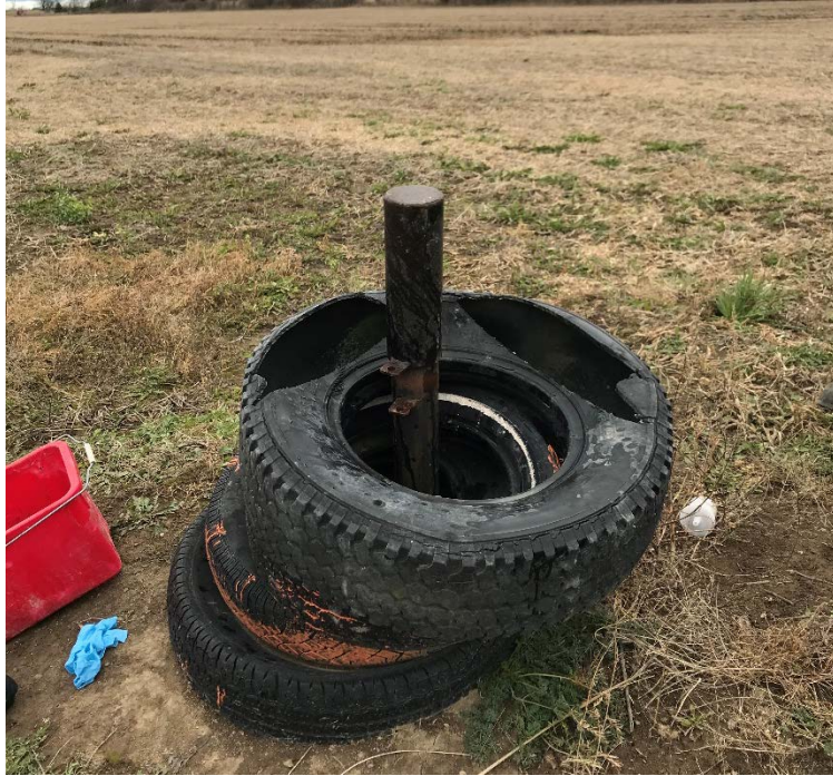
Photo 15: View of monitoring well 91-1 looking southwest.
