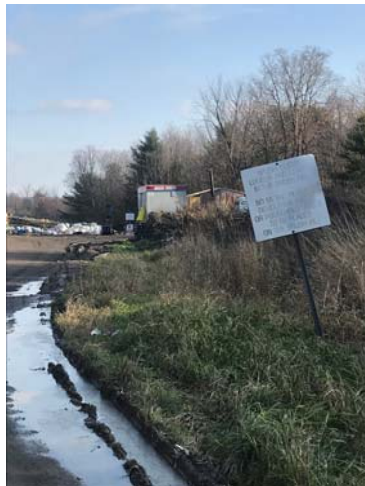
Ponded water at entrance 12-Nov-2018
