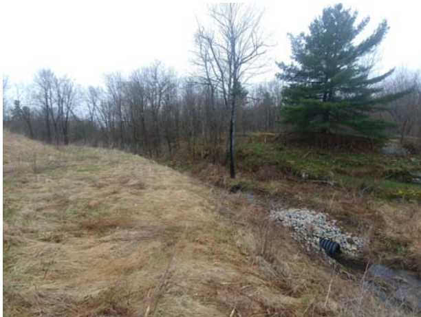
Description: view of the culvert monitored May-2019
