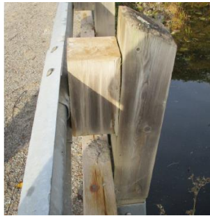
Bridge Railing Wood Post
