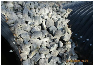
Riprap on Embankment Spacing Between Two Culvert Barrels
